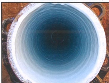
The seamless 1.2 mm epoxy resin coating eliminates corrosion and tuberculation, prevents their recurrence, restores water quality, and optimizes the C-factor (hydraulic efficiency).
